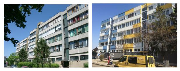
The old curtain walls of the staircases were changed to insulated plastic structure and they were repositioned to reduce the formation of thermal bridges so the new structure has been installed to the outer facade plane.
