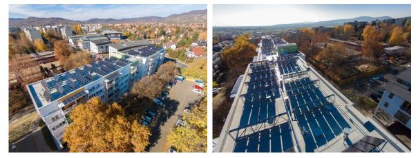
Cogeneration heat and electricity production with 163 pieces of PV/T modules were installed on steel support structures. The total area of the panels is 223,31 m<sup>2</sup>, they will be able to provide up to 30,97 kWp electricity. The produced hot water of the hybrid collectors reduce the DHW consumption of the residential building.
