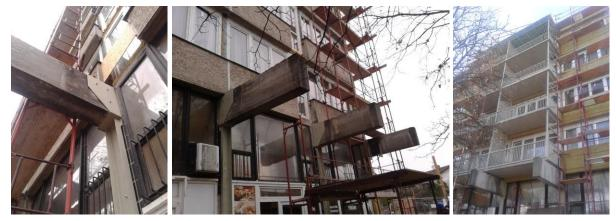
The newly established balconies used to support the existing and remaining reinforced concrete consoles. The four-storey balconies based on the brackets strengthened with steel structure. The balcony plates are prefabricated elements, which were put in place after the completion of the steel frames.
