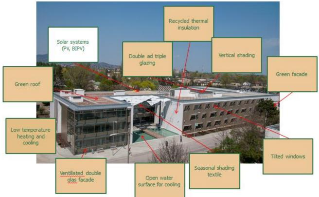
The building is built according to the rules of <u>bioclimatic design</u>. The <u>roof insulation</u> is completed using recycled polystyrene. It is an innovative solution that the EPS insulation boards and the polystyrene part of the light-weight concrete made from recycled material.
