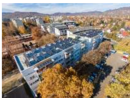
Picture 4 Condominium with photovoltaic thermal panels @PIME'S Concerto project
