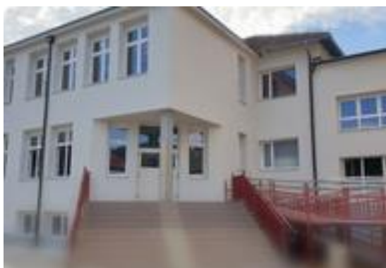
Picture 41.: Elementary school Rada Robiča - during the renovation
