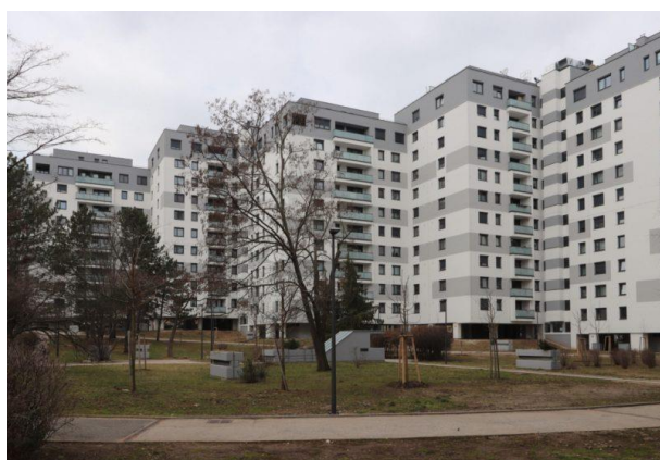
Picture 8: Buildings Freshly Renovated ©GSD
