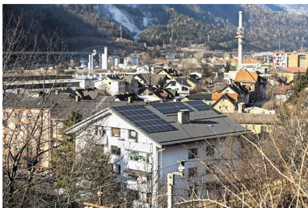
Picture 46: PV panels on the multi-apartment building in Jesenice
