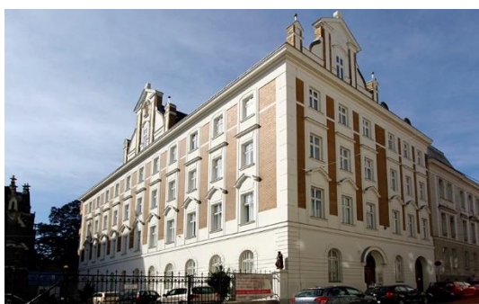
Picture 5: Monastery Building After Renovation @Schöberl & Pöll GmbH
