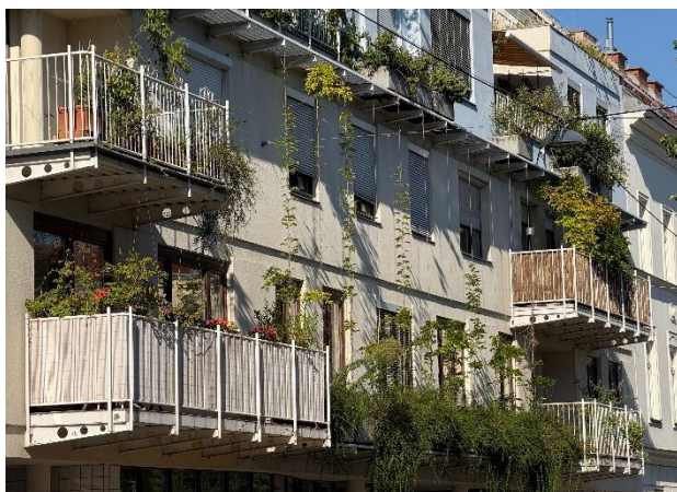
Picture 4: Green Façade Geblergasse Author: @ Isabel Mühlbauer
