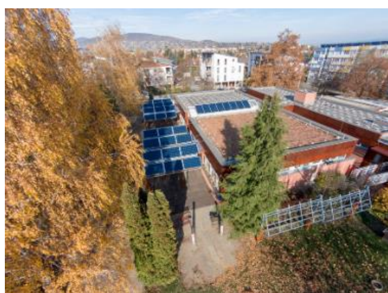
Picture 30: Püspökmajor Kindergarten building after renovation
