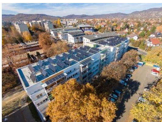
Picture 17: Condominium with photovoltaic thermal panels @PIME'S Concerto project
