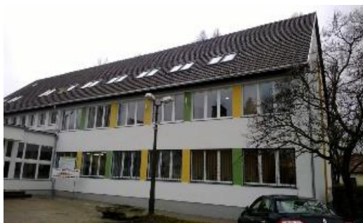
Picture 28: After the refurbishment @PIME'S Concerto project
