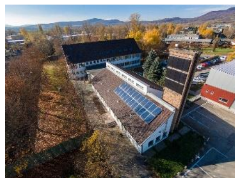
Picture 29: VSZ Zrt. building with PV/T system @PIME'S Concerto project
