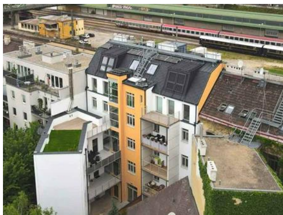
Picture 7: Courtyard View After Renovation ©Graf Holztechnik
