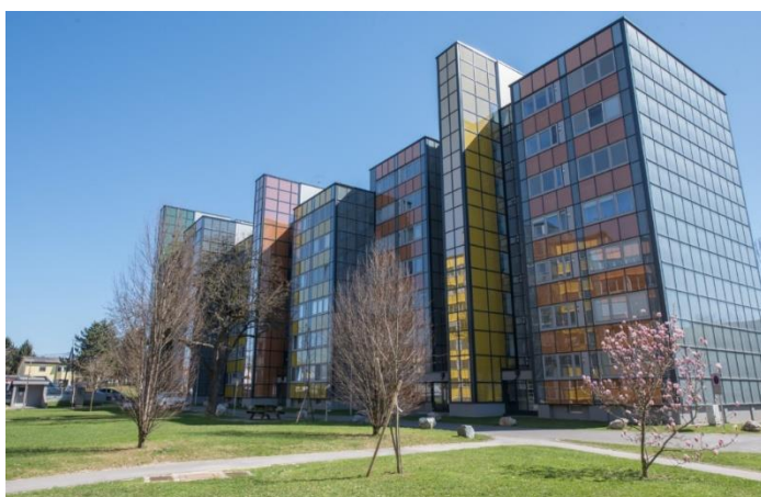
Picture 3: New Façade Elements, ©GAP Solution GmbH
