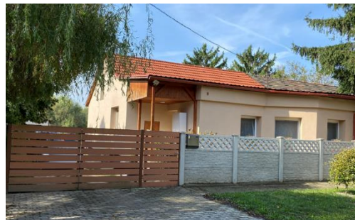
Picture 25: House with insulation and new windows @ with the building owner's permission
