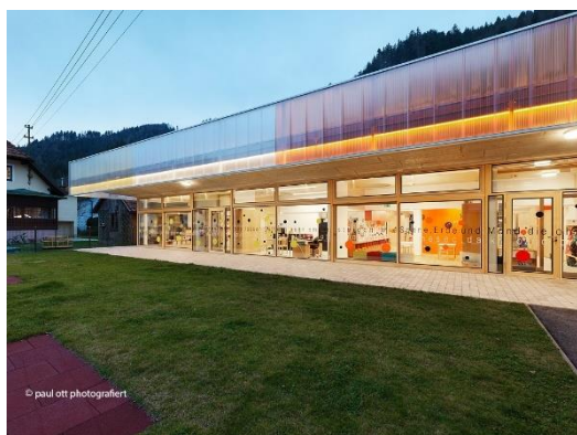
Picture 12: Kindergarten Eisenkappel © Paul Ott
