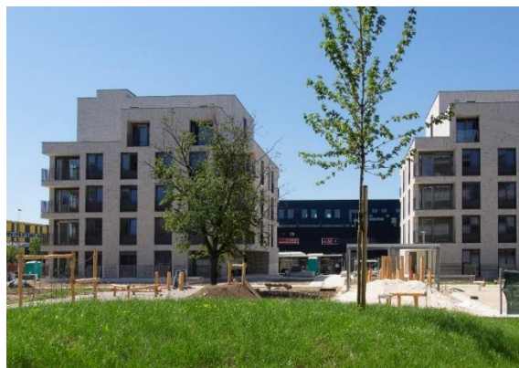
Picture 53.: Apartment bloks at Zvezna ulica, Photo: Gužič Trplan architects
