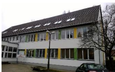
Picture 27: After the refurbishment @PIME'S Concerto project
