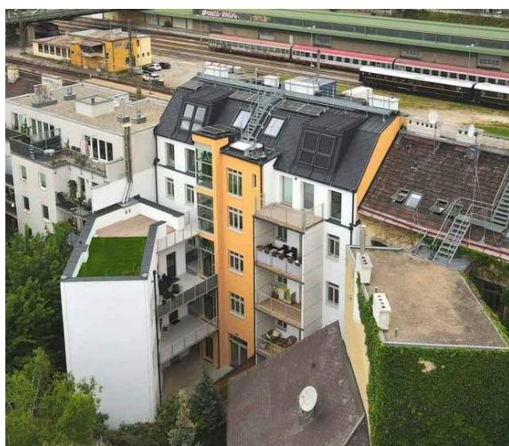
Picture 7: Courtyard View After Renovation, ©Graf Holztechnik
