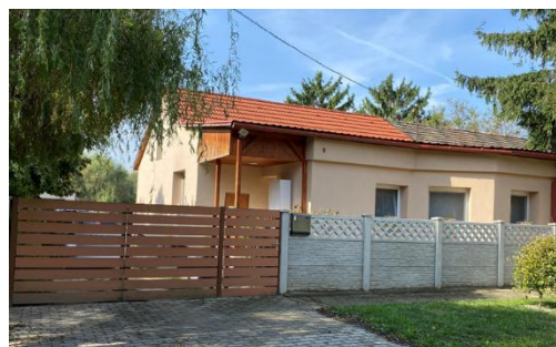
Picture 24: House with insulation and new windows
