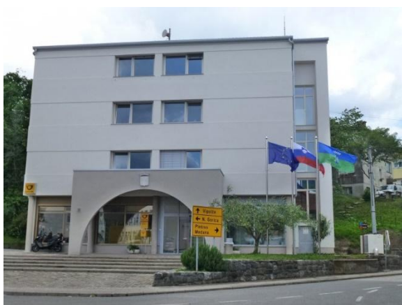
Picture 44: Brda municipal buildings, source: https://www.robin.si/lokalne-novice/briska-obcinska-proracuna-za-leti-2024-in-2025-se-naprej-med-najvisjimi-v-zgodovini-obcine-brda/
