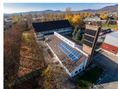
Picture 28: VSZ Zrt. building with PV/T system @PIME'S Concerto project
