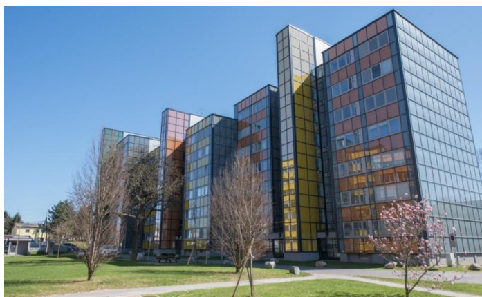
Picture 3: New Façade Elements, ©GAP Solution GmbH
