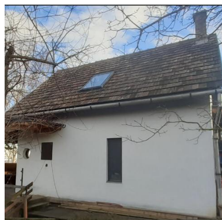
Picture 25: House with new windows
