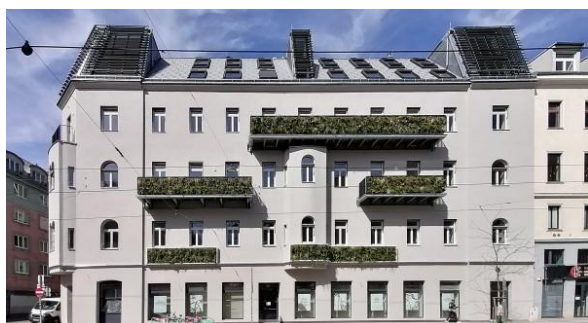
Picture 6: Kauergasse 2 After Renovation ©Trimmel Wall Architekten
