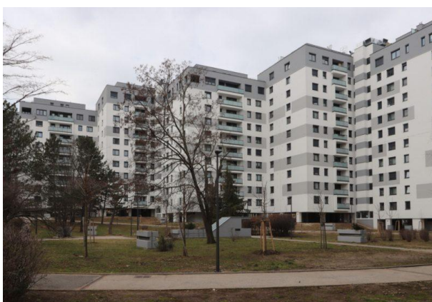
Picture 8: Buildings Freshly Renovated ©GSD
