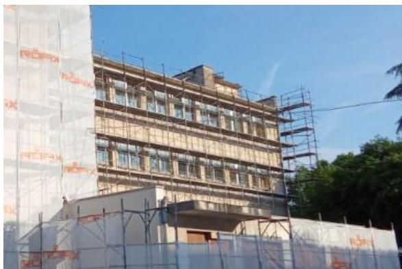
Picture 45: School centre Nova Gorica
