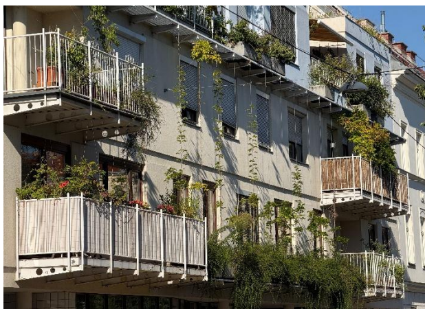
Picture 4: Green Façade Geblergasse Author: @ Isabel Mühlbauer
