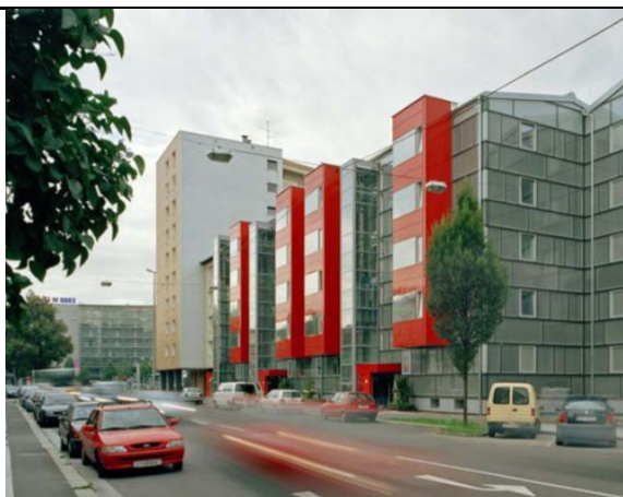
Picture 1: Front Side Apartment Building ©Gemeinnützige Industrie-Wohnungs-AG
