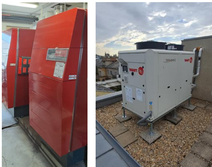
Picture 22: New gas boiler and central cooling system @ Árpád Petrovsky, condominium manager
