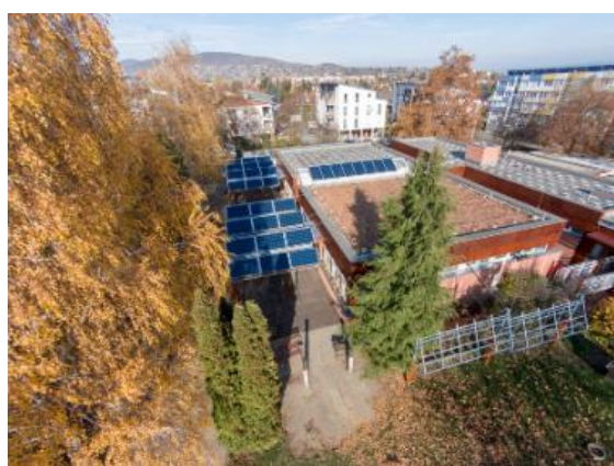
Picture 30: Püspökmajor Kindergarten building after renovation @PIME'S Concerto project
