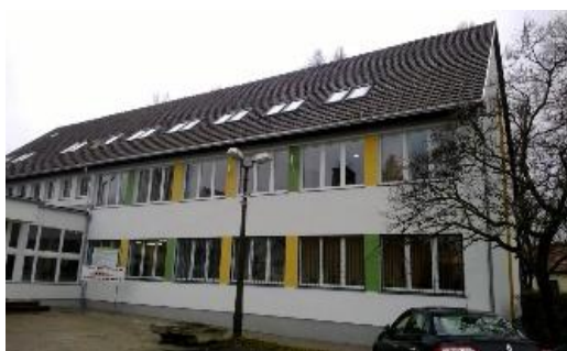
Picture 28: After the refurbishment @PIME'S Concerto project
