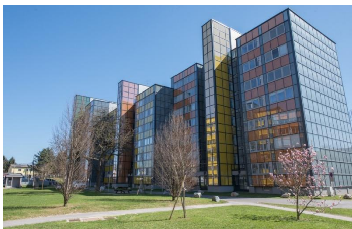
Picture 3: New Façade Elements, ©GAP Solution GmbH
