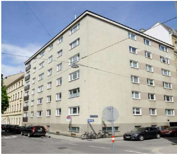
Picture 16.: Before renovation @ Nussmüller Architekten
